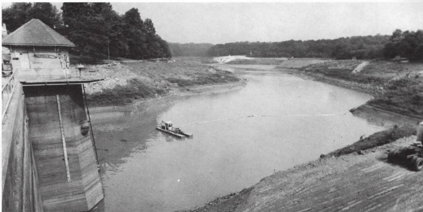
1973 lake restoration after Hurricane Agnes shows the Mud Cat dredge pumping silt into an up-lake decanting basin which is now under water preparatory to major surgery on the dam to install the Bascule Gate.
