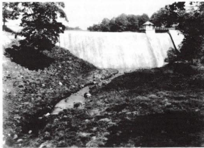
Completed, the Barcroft Dam supplied water to the City of Alexandria. Water company employees released water through underflow pipes. It flowed downstream and was recaptured at Duke Street in Alexandria and stored in a reservoir. (1929)
