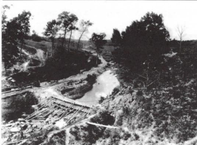
In 1913, the Piedmont Construction Company began building the Barcroft Dam by laying railroad tracks in the Holmes Run valley to transport rock for the dam and building a makeshift coffer dam to control stream flow. (September 13, 1913)
