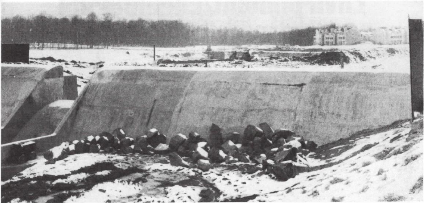
Reservoir 2A's gravity concrete dam nearing completion with the now-being-excavated lake in the background.
